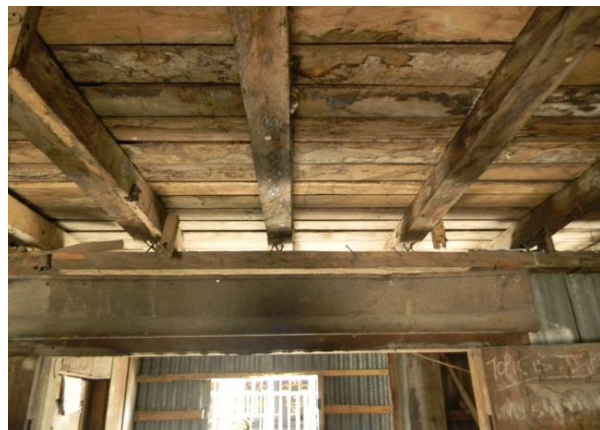
Figure 9: suspended timber floor Bobmanuel house Abonema Source: Author (2016)
