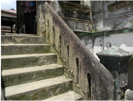
Figure 13: Ornamented staircase Source: Author (2022)
