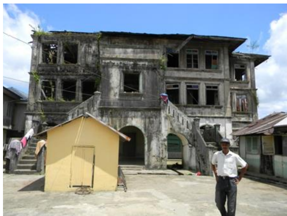
Figure 22: double-sided staircase to upper floor entrance Source: Author (2022)
