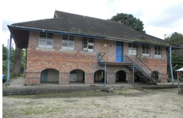
Figure 2: British colonial residence in Degema Source: Author (2022)
