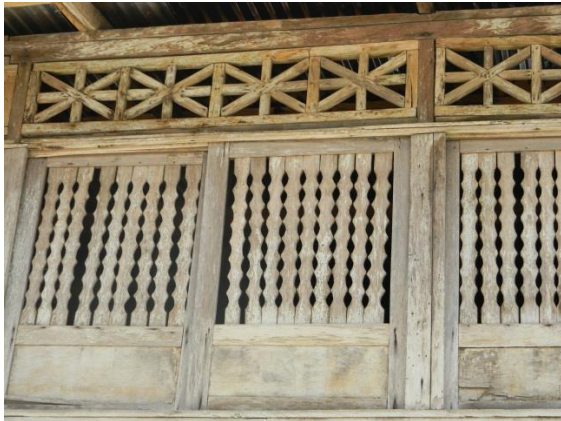
Figure 11: 3-dim timber 'frontal-styled' lintel frame BobManuel house, Abonema Source: Author (2016)
