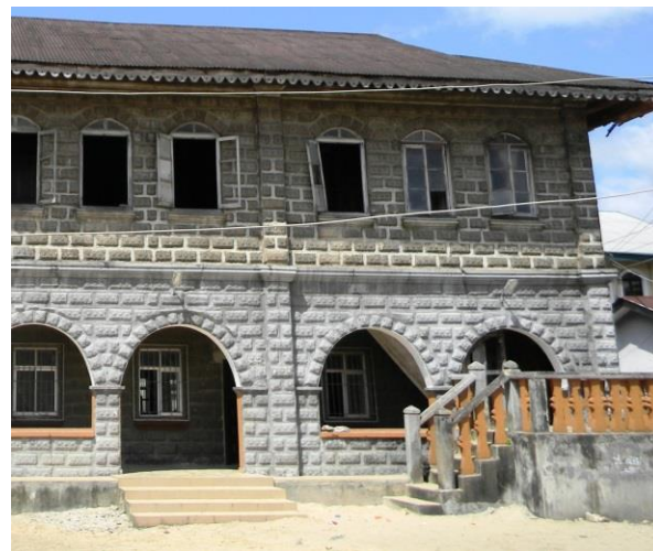
Figure 24: Use of arches and elaborate stairs Source: Author (2022)
