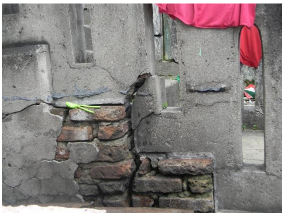
Figure 15: Use of fired bricks rendered over with mortar Source: Author (2022)
