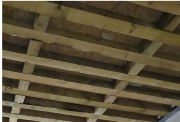
Figure 8: Restored suspended timber floor Source: House in Lisbon, Henriques (2020)
